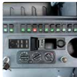
Centralized Instrument Switch Panel
